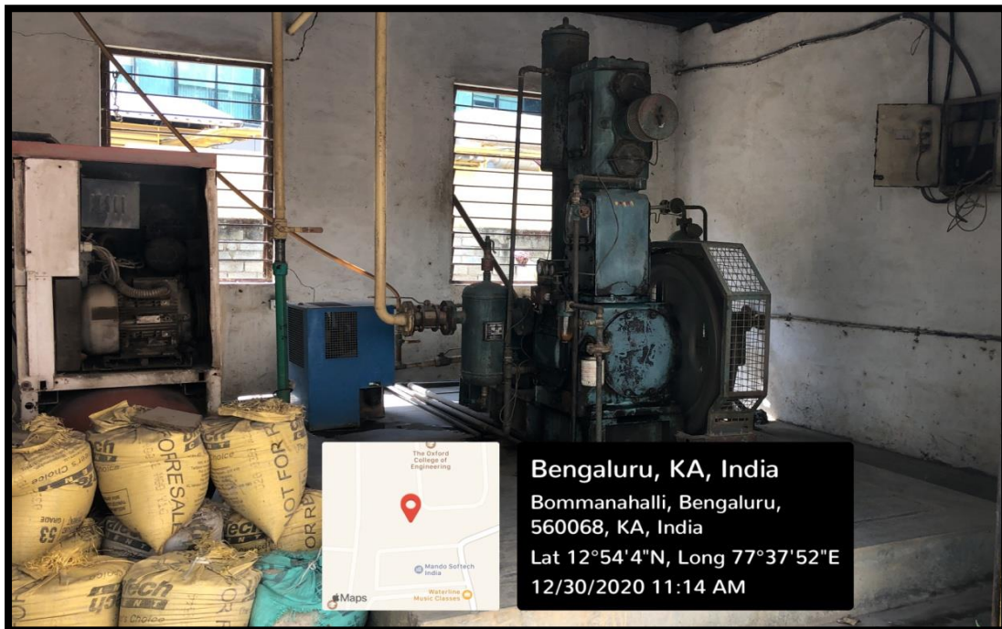
Centralized Compressor for Dental Departments
